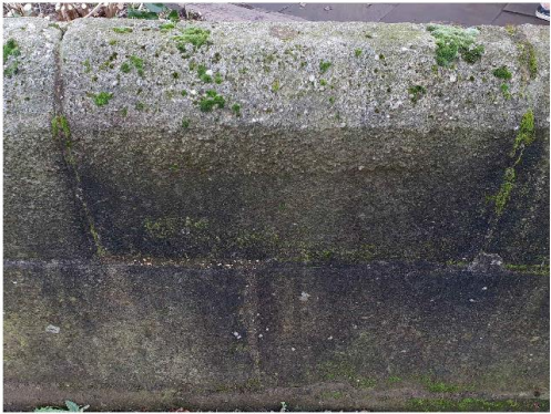
PHOTOGRAPH OF PROPOSED FINISH TO WALL STRENGTHENING
